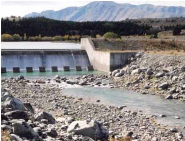
Natural character rating: 10% Key attributes: flow modification, man-made structure
